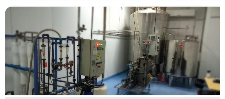
• Equipped with a Pure Water system with 10,000 liter tanks and loop piping, covering an area of more than 7,000 square meters
